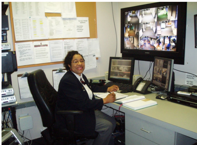
Above: Martha Rogers monitors the security cameras from the control room at the Chatham County Courthouse.
