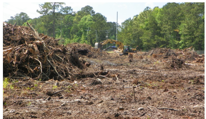
Above: Construction crews cut down dozens of trees near the booking area to make way for a new video visitation center.
