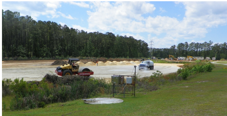
Left: Most of the construction will take place on the south side of the existing jail. Contractors say the expansion project will take about 30 months to complete.
